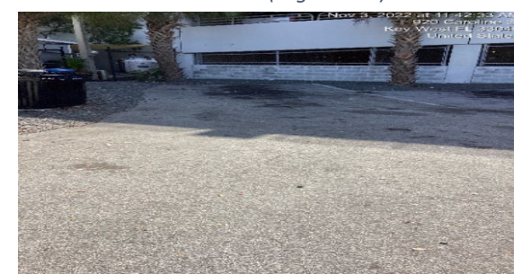
Raveled and cracked paving
